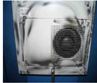
1,500 watt wall-mounted cooling units/soiled by graphite dust from the air
