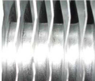
1,500 watt wall-mounted cooling units/soiled by graphite dust from the air
