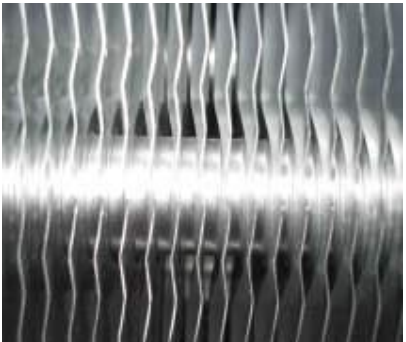
1,500 watt wall-mounted cooling units/soiled by graphite dust from the air
