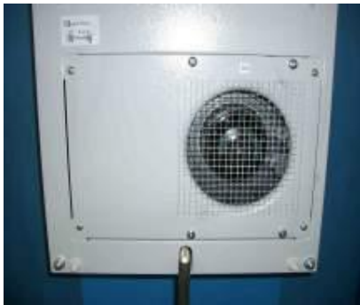
1,500 watt wall-mounted cooling units/soiled by graphite dust from the air
