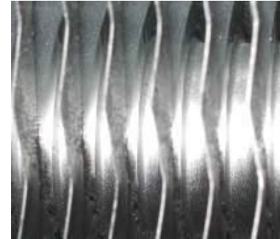
1,500 watt wall-mounted cooling units/soiled by graphite dust from the air
