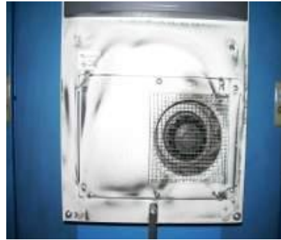
1,500 watt wall-mounted cooling units/soiled by graphite dust from the air
